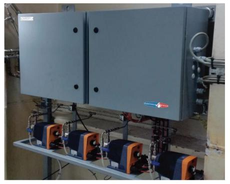
blowdown: improving control, saving energy and chemicals. In addition the system provides remote monitoring with PC-based Data Management software, with data logging, analysis and diagnostic capabilities with alarms to ensure that the close control achieved does not degrade over time.
