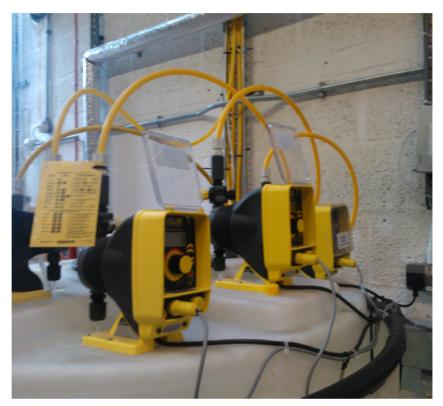
The quality of feedwater for any boiler has to be controlled, broadly in line with steam output. Sulphite or DEHA to treat the oxygen content, caustic for pH control and a touch of phosphate for hardness control.
