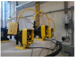
Diaphragm driven metering pumps have been the stalwart choice for dosing treatment chemicals ever since the Economic Boiler replaced the Lancashire and Cornish boilers. Once the stroke length and stroke rate have been manually adjusted they are left to quietly get on with dosing chemicals with minimum intervention. To err on the side of caution, they
