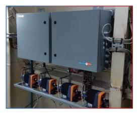
The **C4S-AQ300** is a fully automated water monitoring and control system which scrutinises boiler feedwater to ensure chemical dosing is aligned to real-time water quality and the demands of the boiler, protecting the water system and steam plant 24 hours a day.
